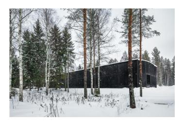
The 1056 square metre black warehouse of the Finnish Kyrö Distillery is located in the middle of the forest and at first glance appears to be boarded up with old, charred wooden planks. The façade of the barrel warehouse is inspired by the traditional wooden barns.
